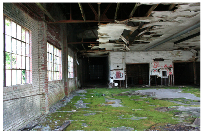
Right: Interior prior to renovation.
