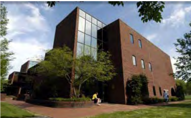
COLE COMPLEX AHU Replacement
