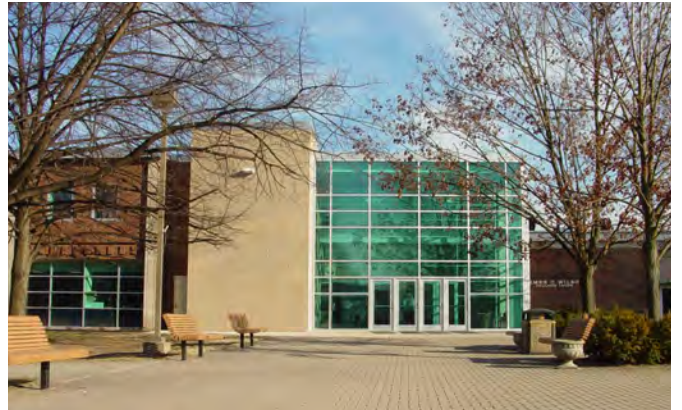
JAMES C. WILSON STUDENT UNION HVAC Replacement
