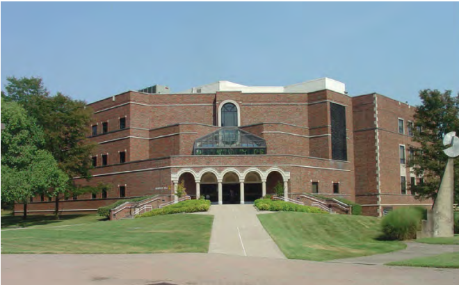
HAMBLIN HALL HVAC Replacement
