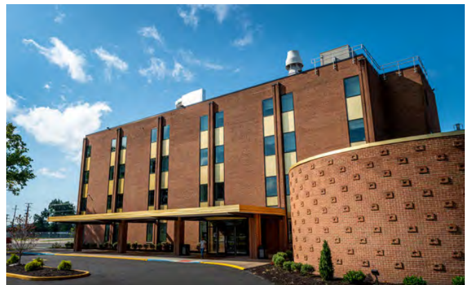
F. RAY POWERS RESEARCH LAB Renovations
