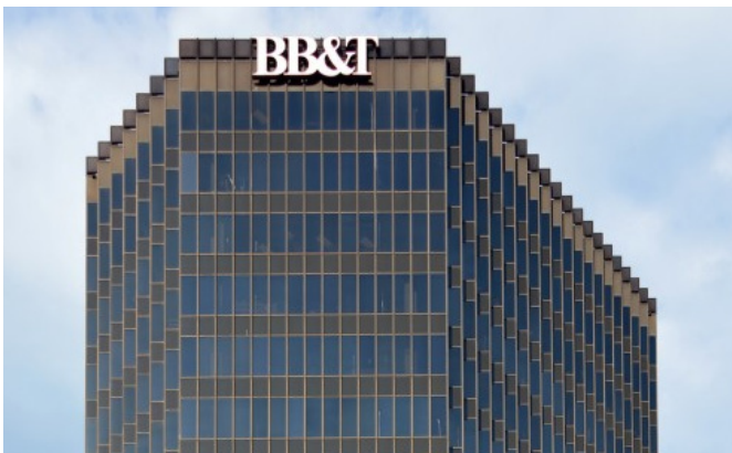
BB&T BANK OFFICE TOWER Elevator Modernization
