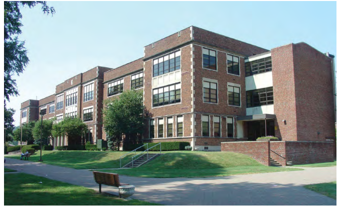
FERRELL HALL HVAC Replacement
