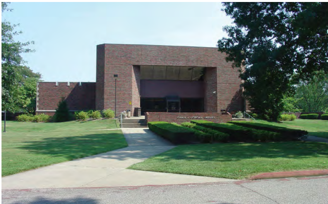
DRAIN JORDAN LIBRARY HVAC Replacement
