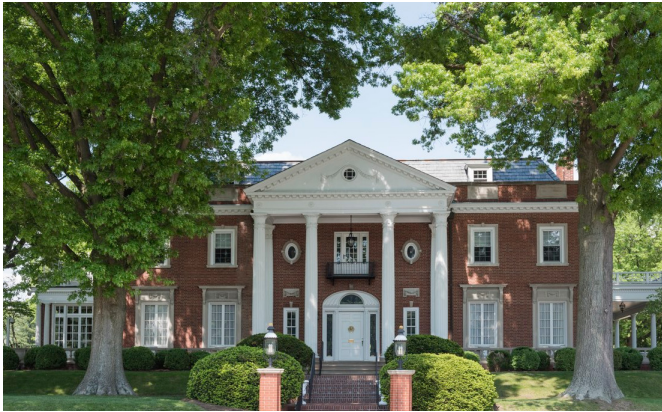
WV GOVERNOR'S MANSION Elevator Modernization
