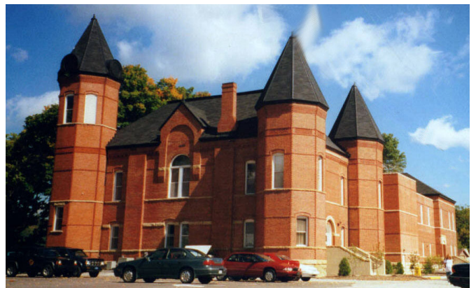
PUTNAM COUNTY COURTHOUSE Roof Replacement
