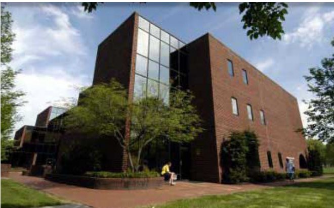
COLE COMPLEX AHU Replacement
