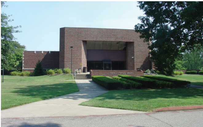
DRAIN JORDAN LIBRARY HVAC Replacement
