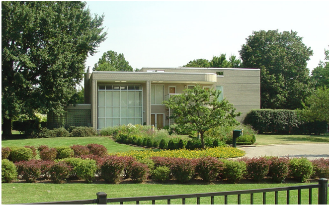
PRESIDENT'S HOUSE Roof Replacement & Arbor Design
