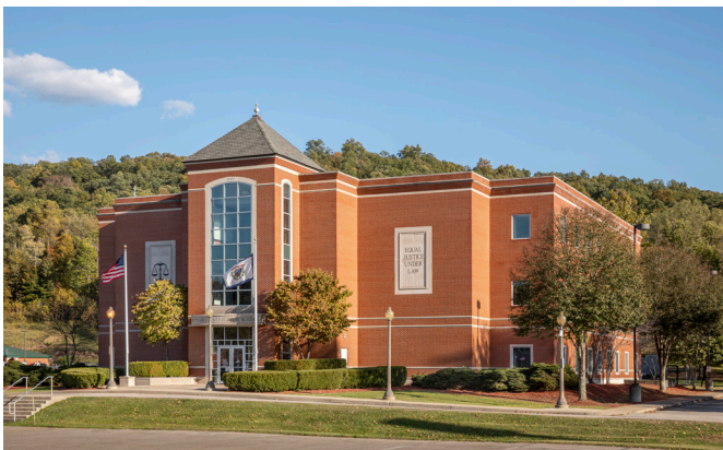
PUTNAM COUNTY JUDICIAL BUILDING Roof Replacement
