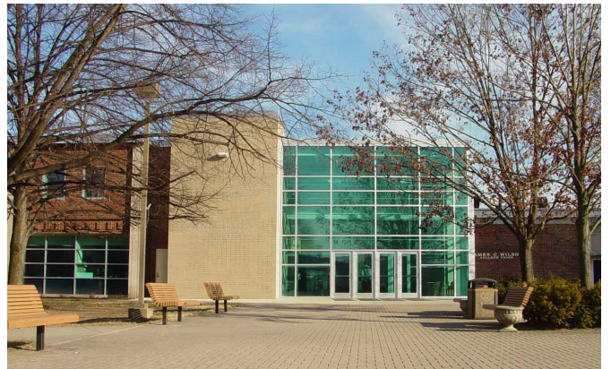
JAMES C. WILSON STUDENT UNION HVAC Replacement
