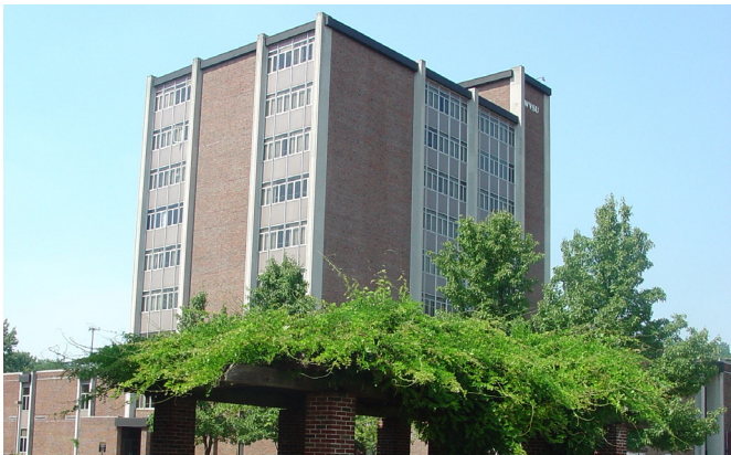
WALLACE HALL Boiler Replacement
