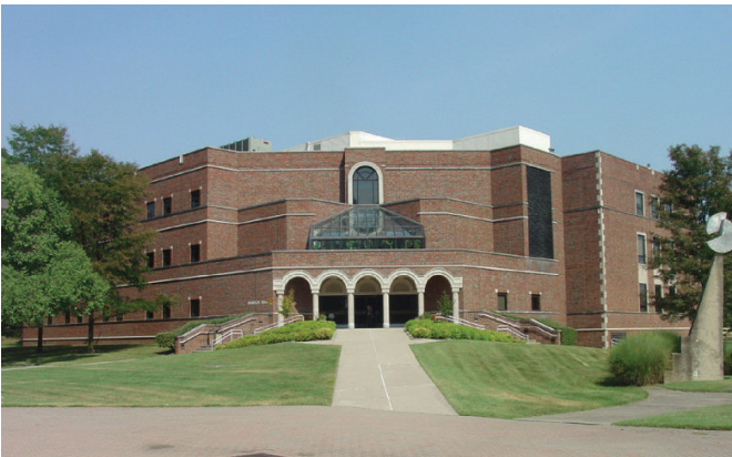
HAMBLIN HALL HVAC Replacement
