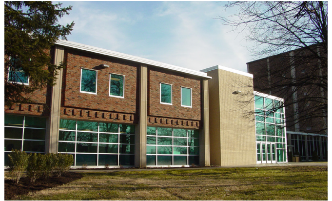
JAMES C. WILSON STUDENT UNION Roof Replacement
