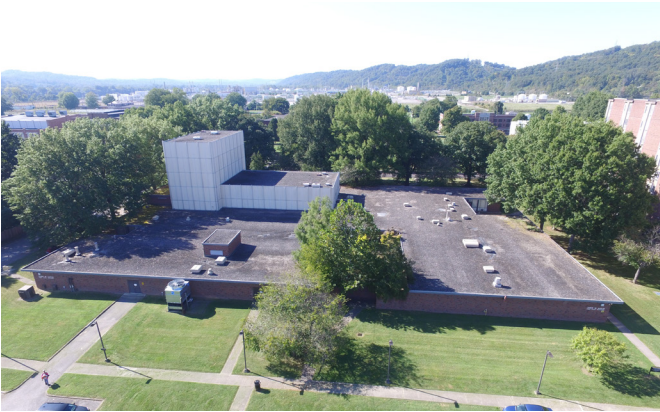
DAVIS FINE ARTS CENTER Roof Replacement Study
