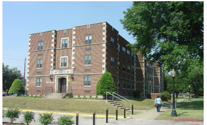
HILL HALL Steam Boiler
