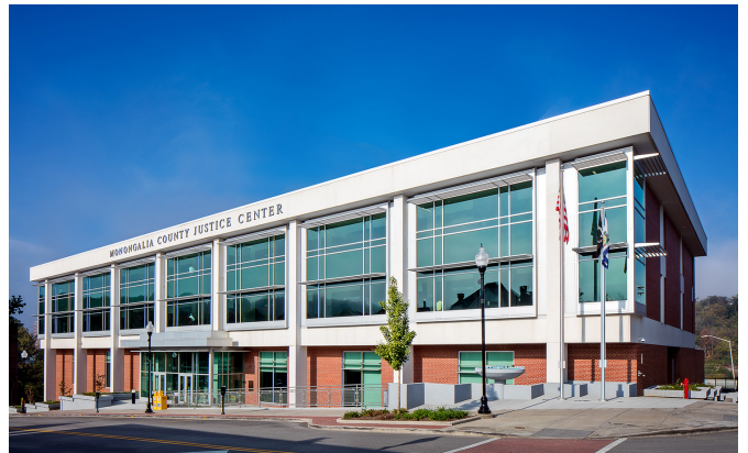
MONONGALIA COUNTY JUSTICE CENTER Roof Replacement
