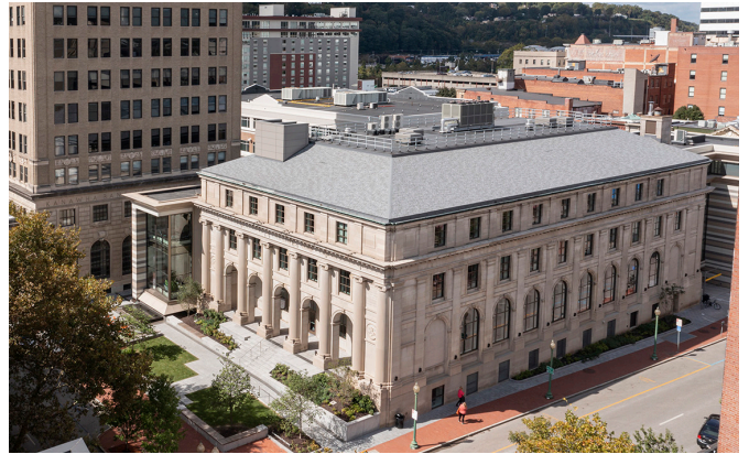
KANAWHA COUNTY PUBLIC LIBRARY Roof Replacement
