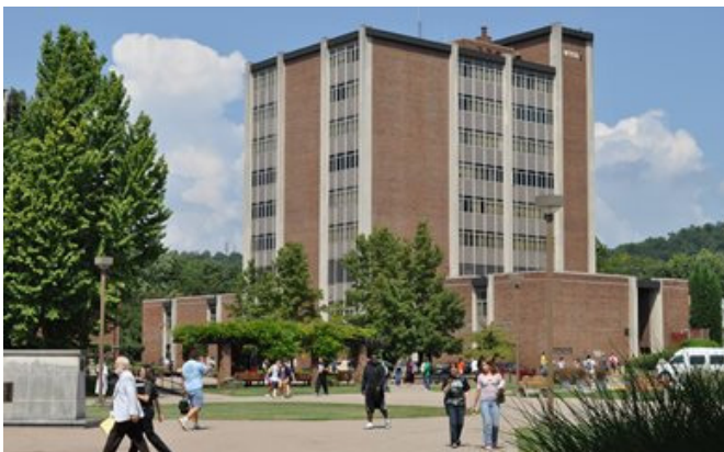
WALLACE HALL Roof Replacement
