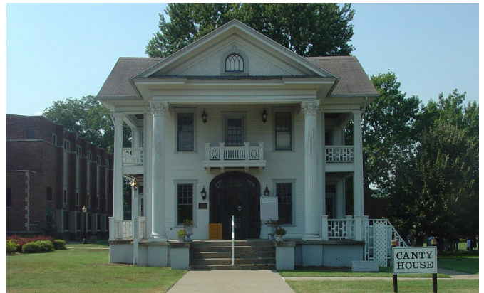
CANTY HOUSE Roof Replacement
