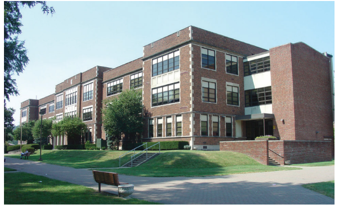
FERRELL HALL HVAC Replacement
