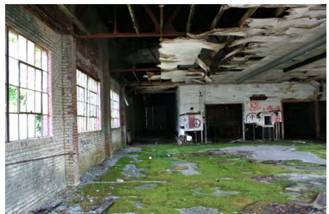
Right: Interior prior to renovation.
