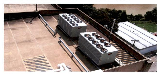
Charleston Coliseum & Convention Center (2015) – Replace entire MEP infrastructure three 1,000 ton chillers and cooling towers, three 8,000 mbh gas condensing boilers, approximately ten VAV AHU's, approximately 10 large single zone VAV AHU's.
