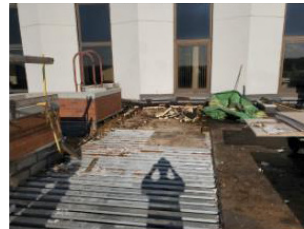
512.20 Decking & Remaining Debris
