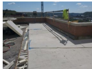
512.20 tapered system, installed cricket, 5 hard board
