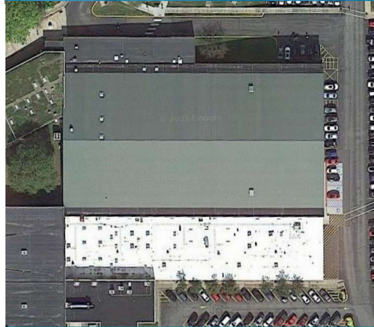
Morrow Field House Roof Replacement
