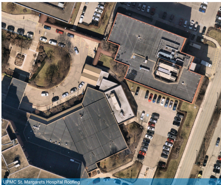
UPMC St. Margarets Hospital Roofing
