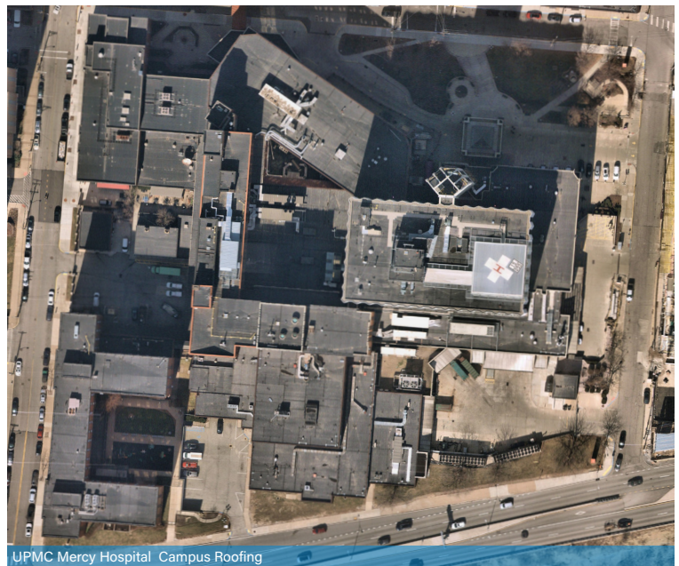
UPMC Mercy Hospital Campus Roofing
