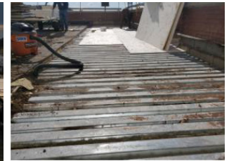
512.20 Dense deck & cleared flutes
