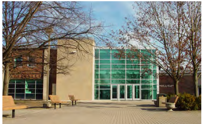
JAMES C. WILSON STUDENT UNION HVAC Replacement
