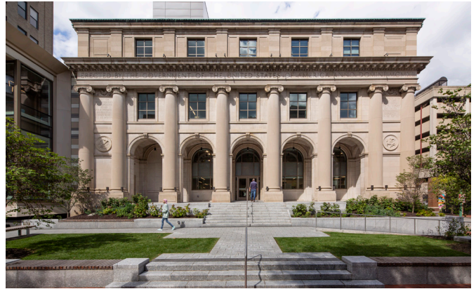
KANAWHA COUNTY PUBLIC LIBRARY Elevator Upgrades
