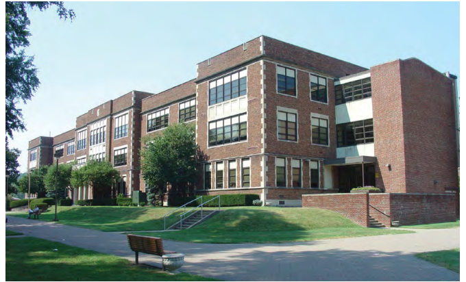
FERRELL HALL HVAC Replacement
