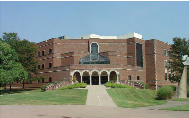
HAMBLIN HALL HVAC Replacement
