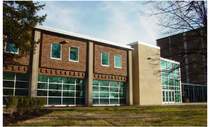
JAMES C. WILSON STUDENT UNION Roof Replacement
