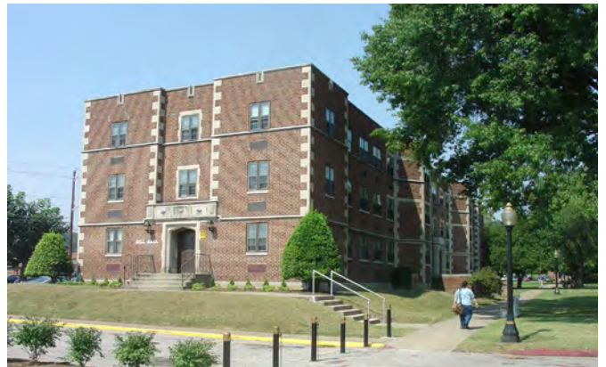
HILL HALL Steam Boiler
