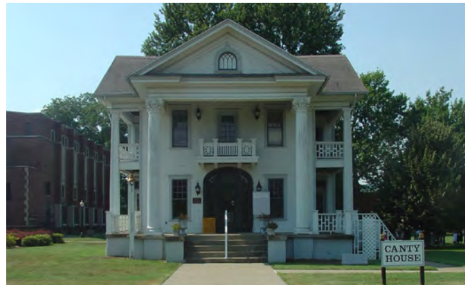
CANTY HOUSE Roof Replacement
