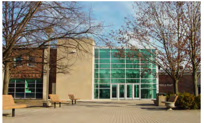
JAMES C. WILSON STUDENT UNION HVAC Replacement
