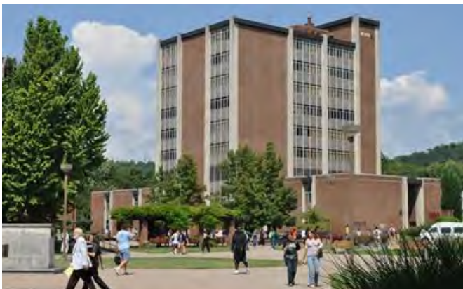
WALLACE HALL Roof Replacement
