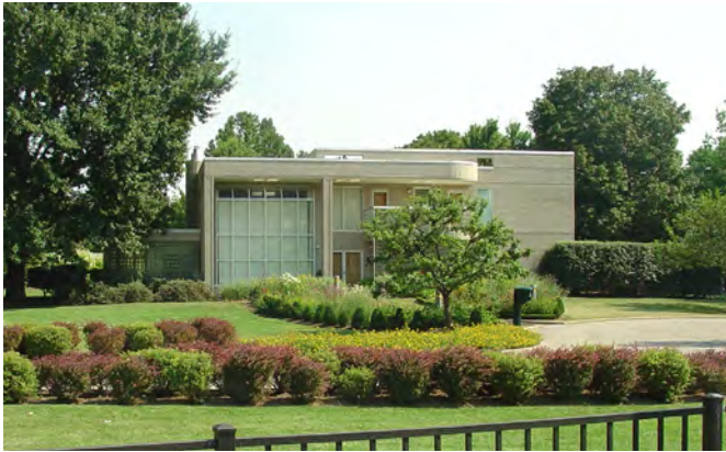
PRESIDENT'S HOUSE Roof Replacement & Arbor Design
