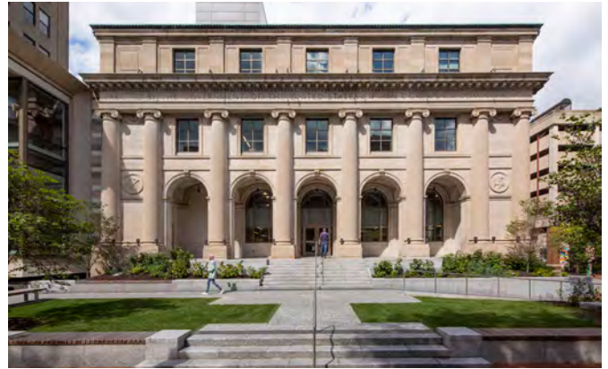
KANAWHA COUNTY PUBLIC LIBRARY Existing Building - New Sprinkler System
