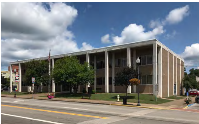
ROANE COUNTY COURTHOUSE Existing Building - New Sprinkler System
