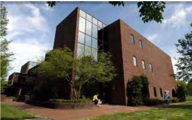
COLE COMPLEX AHU Replacement
