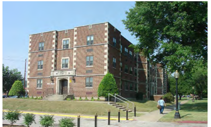
HILL HALL Steam Boiler
