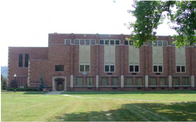
WVSU - FLEMING HALL Existing Building - New Sprinkler System
