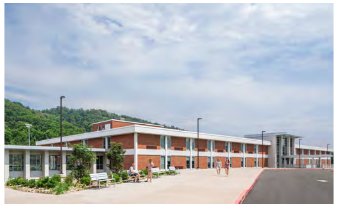
JOHN MARSHALL HIGH SCHOOL Existing Building - New Sprinkler System
