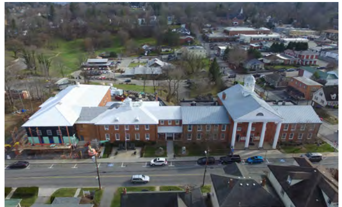
GREENBRIER COUNTY COURTHOUSE Existing Building - New Sprinkler System
