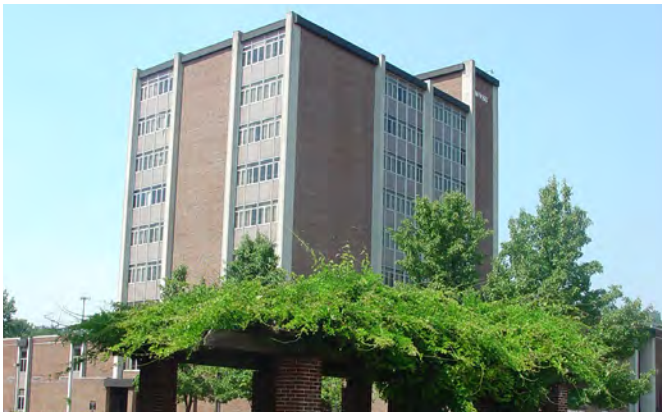
WALLACE HALL Boiler Replacement
