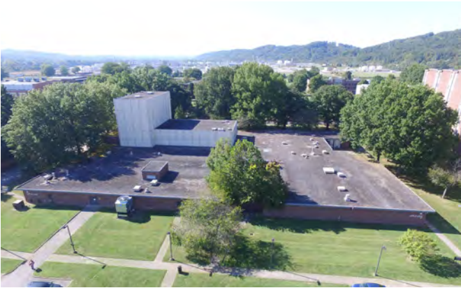
DAVIS FINE ARTS CENTER Roof Replacement Study
